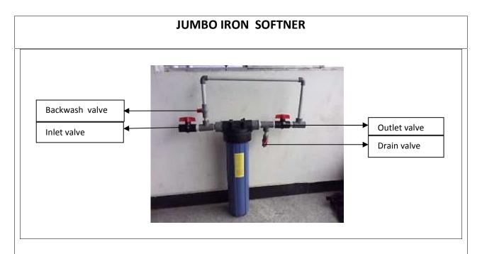
Iron remover system is designed to remove iron from raw water. Iron removal system reduces iron, helps eliminate orange and brown stains in sinks, tubs and other plumbing features, and improves water taste. It also reduces possibility of damage to pipes, and reduces dissolved iron.
